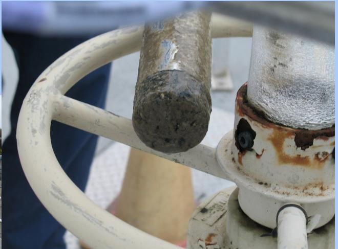
DO meter sensor fouling - requiring frequent cleaning.
