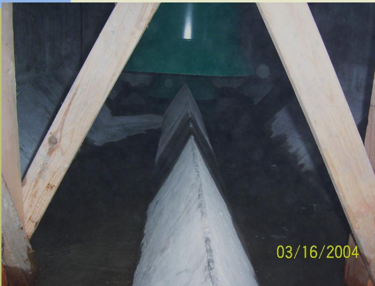
Flow splitter under pump inlet
