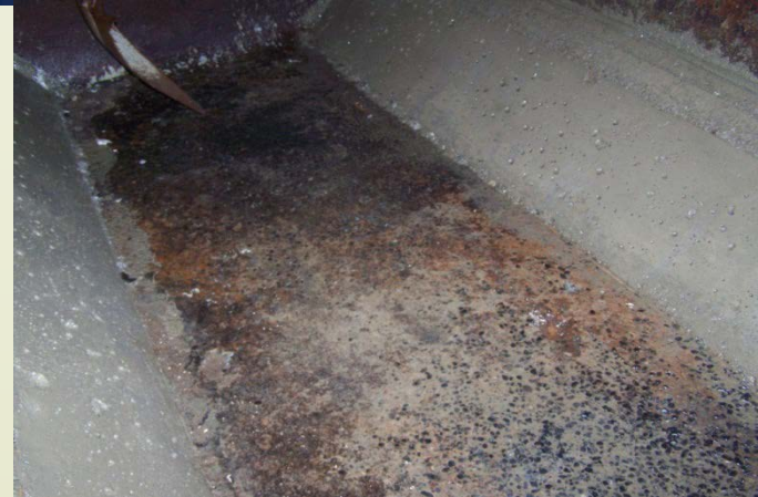
Concrete fillets in corners
