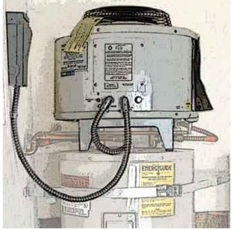
A storage water heater can be converted to a HPWH with an add-on unit, either wall-mounted or sitting on top of the existing tank.
