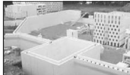
Conventional finishes are applied to suit the building. ICF systems are differentiated by the type of insulation, the shape of the cavity and the method of connecting the insulation layers. The basic cavity shapes of the concrete blocks are flat, grid and post-and-beam. Many, but not all, ICF systems meet the thermal requirements of the *Washington State Energy Code (WSEC)*, see WSEC Tables 6-1 and 6-2.
