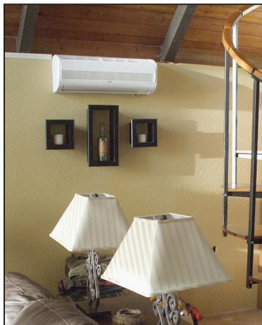
Air handler with blower and heat exchange coil
