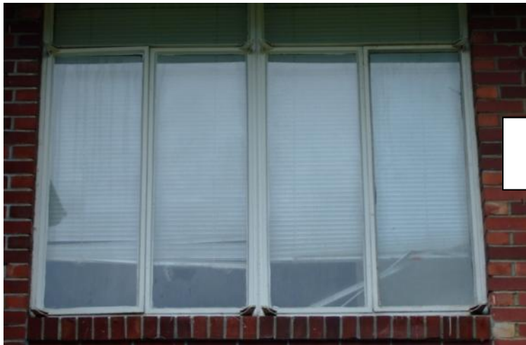
Original single-pane, metal-framed casement windows
