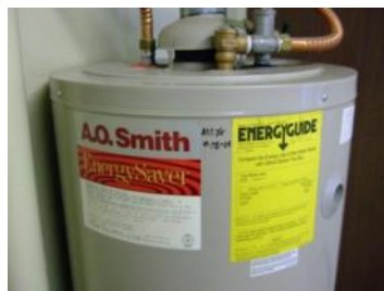
Figure 7b. Typical 0.60 - 0.62 EF natural gas tank water heater
