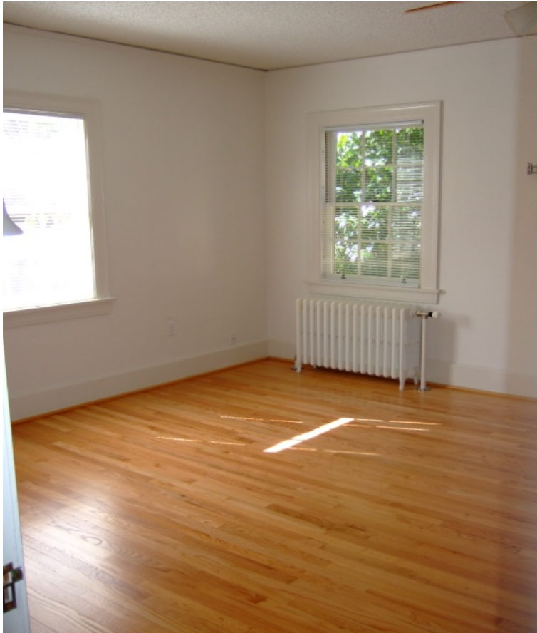
Hydronic radiator typical throughout homes in the historic Broadmoor development
