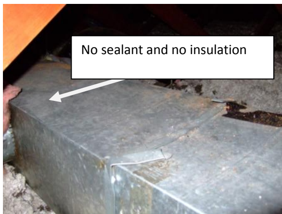
Figure 15a. Typical duct system
