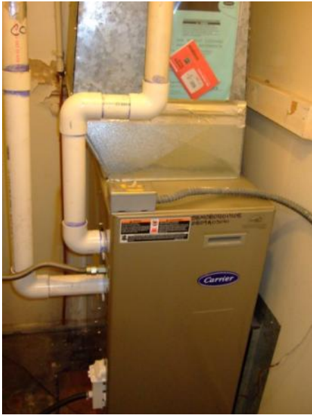
Figure 6a. Typical sealed combustion natural gas furnace
