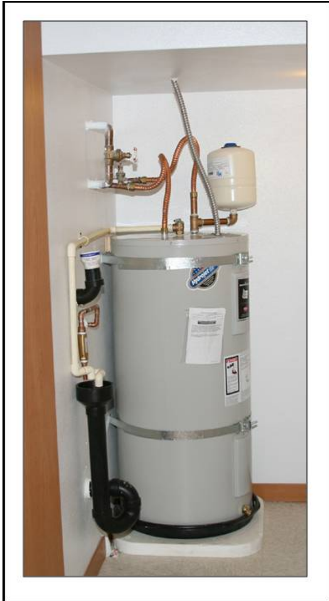
Figure 16. Photo of Typical Water Heater Installed in Conditioned Space
