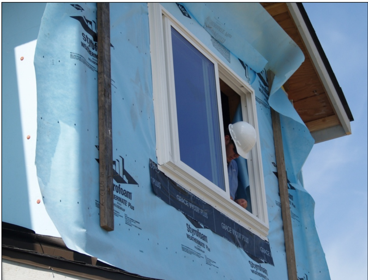
Figure 8. Photo of High Performance Window Flashing
