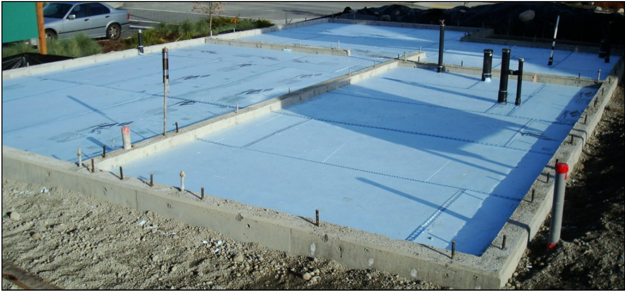
Figure 7. Photo of 2" R-10 XPS Installed Under a Slab at High Point
