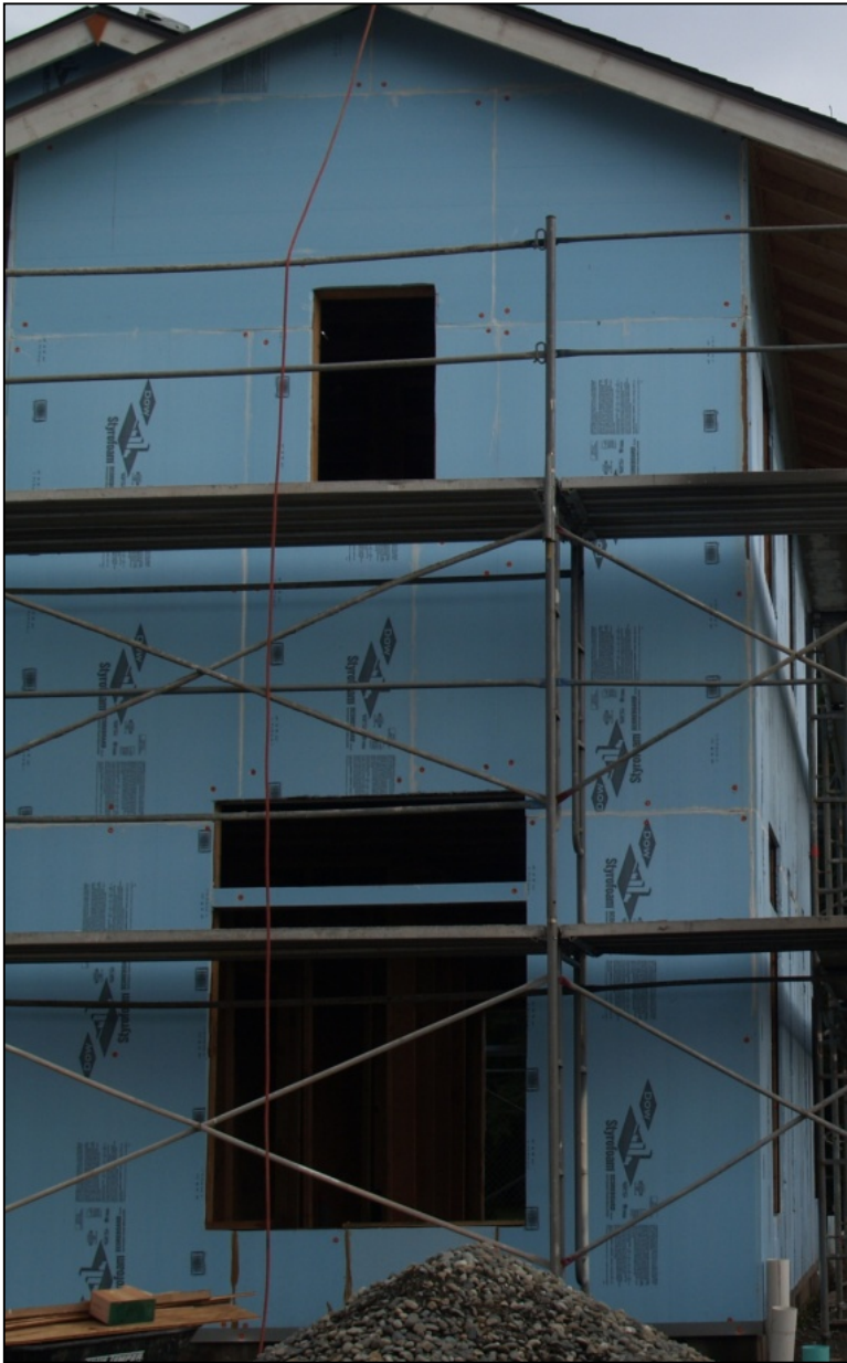
Figure 3. Photo of Rigid Foam Board Installed on the Exterior of the Wall Assembly
