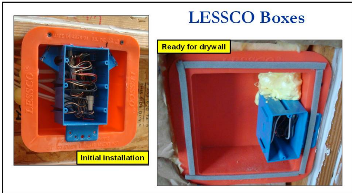
Figure 1. Photo of a Lessco Box Used in Air Sealing Electrical Boxes
