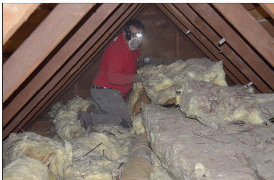
CEEP contractor insulating a residential attic.
