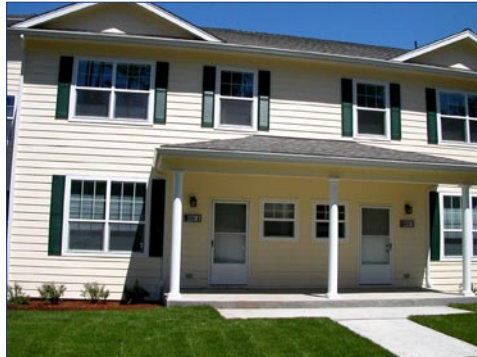
Figure 1. Equity Residential and Champion Homes have started construction on 864 energy efficient homes on the Ft. Lewis Army Base in Washington State.
