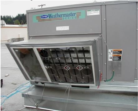
Figure B1. Flow Grid Installed on Outdoor Intake Hood
