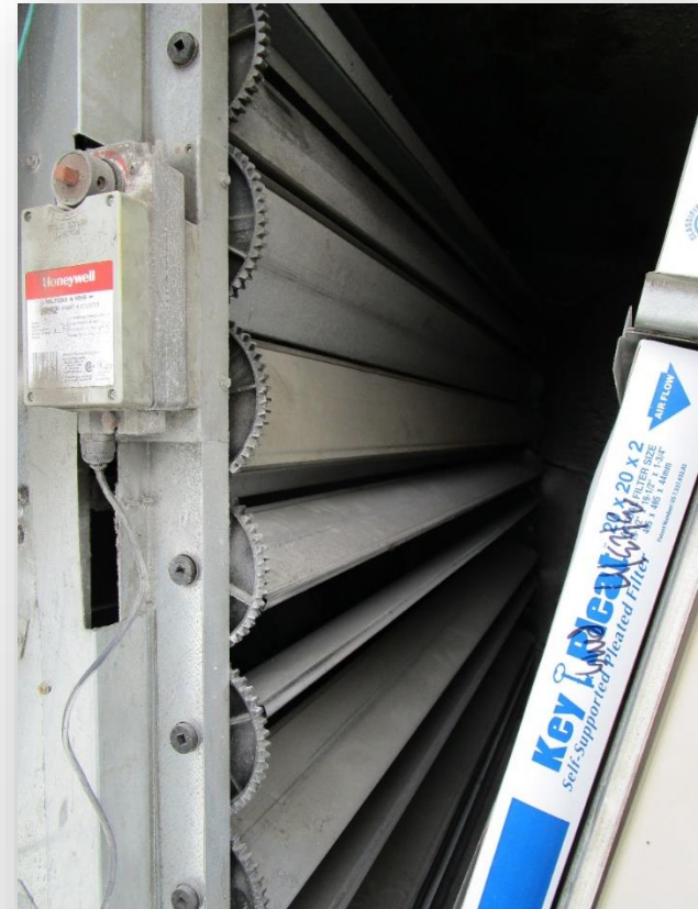
Economizer dampers and actuators
