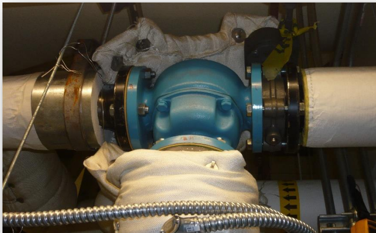
Valve Insulation Jacket Removed
