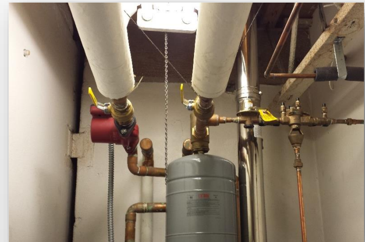
Pipe Insulation Not Replaced After Expansion Tank Replacement
