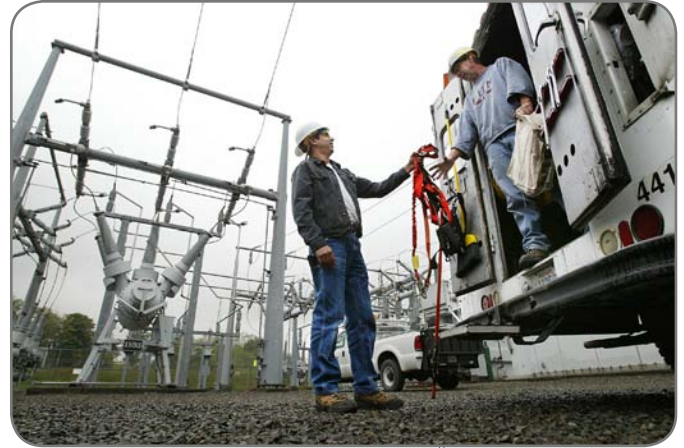
Workers at Substation 10
