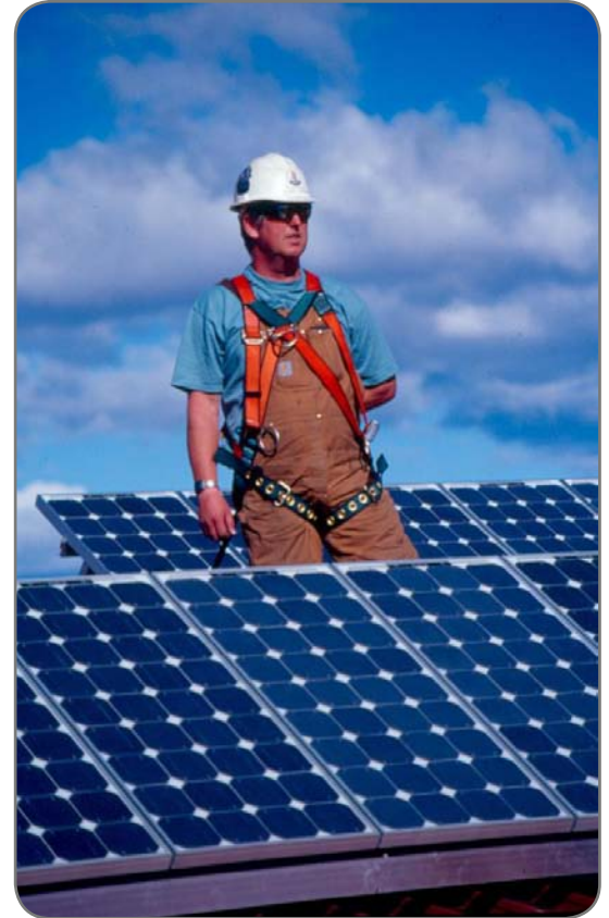
Solar panels on the roof of Wenatchee Valley College Photo courtesy of Chelan County PUD
