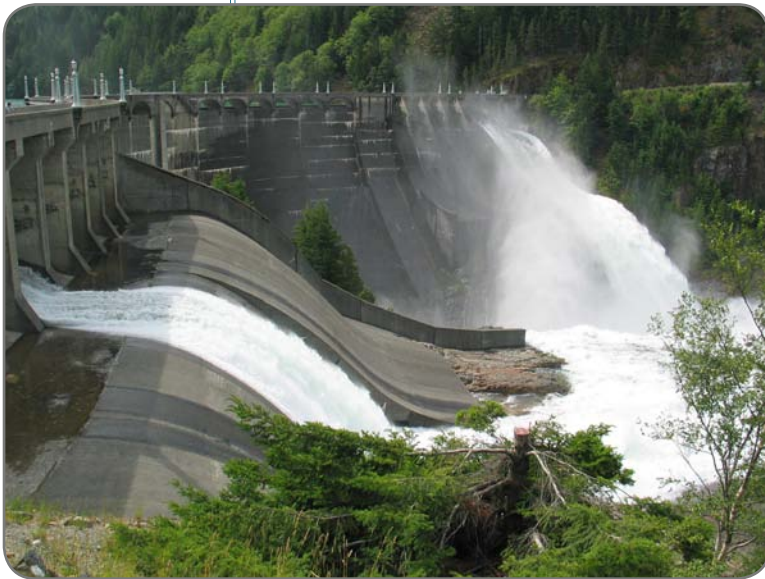
Diablo Canyon Dam Spillway
