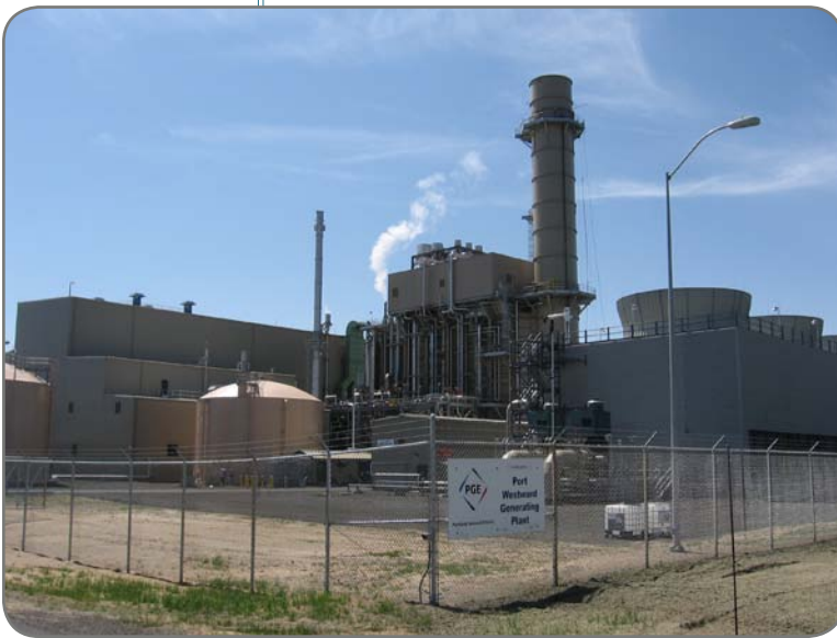
Port Westward Generating Plant
