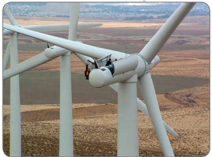
Workers service a wind turbine at the Nine Mile Canyon Facility
