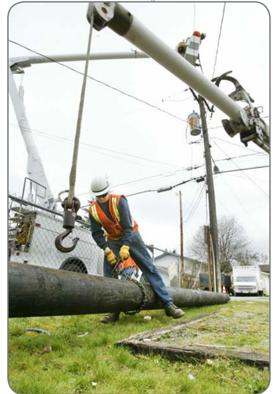
Setting a Pole
