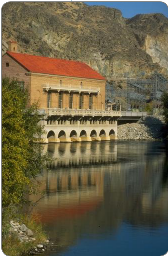
Chelan power house
