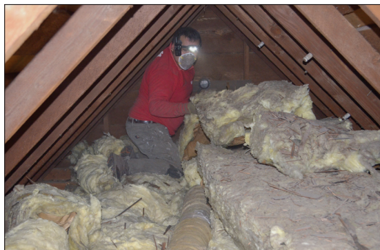
CEEP contractor insulating a residential attic.
