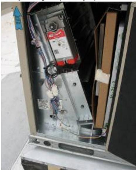
The economizer modulates exhaust air, return air and outside air dampers to maintain the mixed air temperature at its setpoint (around 60°F.) The action of the outside air damper and relief damper, if there is one, should always be opposite that of the return air damper. When the outside air is cool enough to cool the building (about 60°F or less) and there is a call for cooling, the
