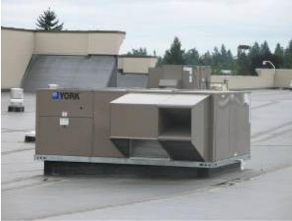
In order for the economizer to function, the HVAC system needs to be on and in the first stage of cooling. This is most easily accomplished by connecting a jumper wire at the terminal strip. **This should be done by the installer in accordance with the manufacturer's recommendations.** If the outdoor temperature is below 60°F, the unit's outside air damper should slowly modulate open. If it doesn't, try cooling the outside air sensor with some ice in a plastic bag or by spraying it with
