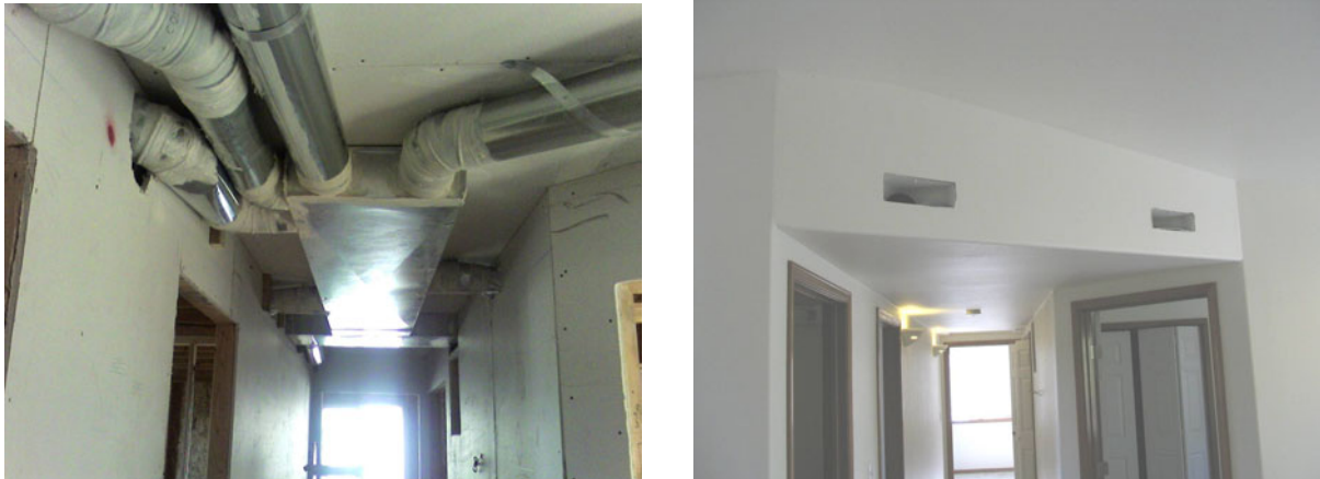
Figure 1. Habitat for Humanity, Moses Lake - Duct Chase Pre- and Post-Drywall
