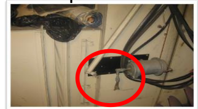
Disconnected Damper
