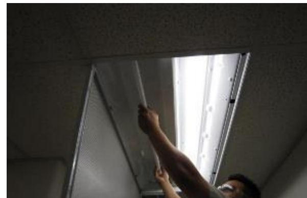
Replace 32-watt T8 lamps with 28 or 25-watt lamps
