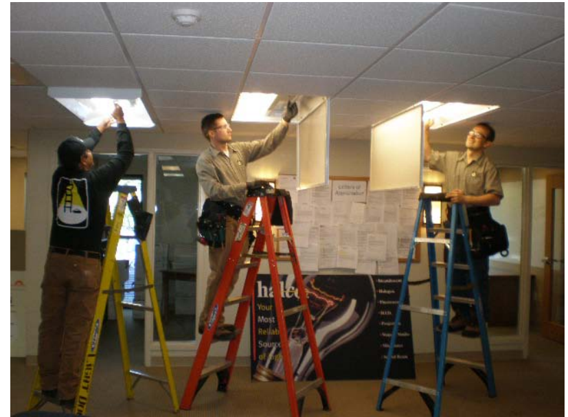
Quick Lighting retrofit in progress
