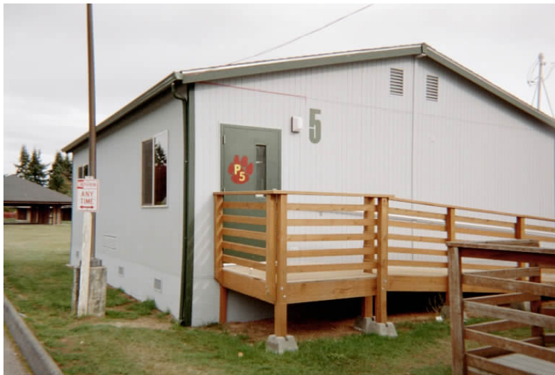
Figure 1: Energy Efficient Portable Classroom – Pinewood Elementary School, Marysville, Washington
