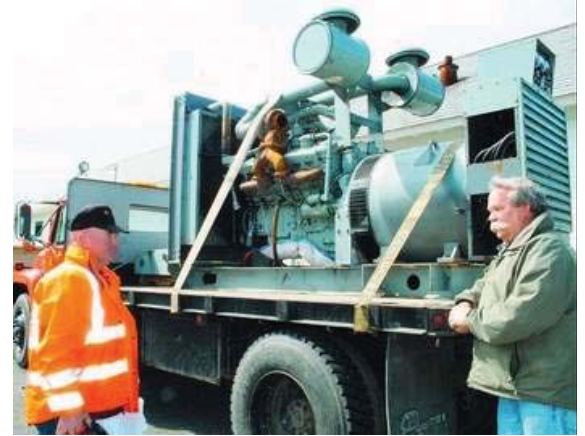
Jay Ketchum, owner of Affordable Crane of Agnew, left, talks to Russ Hendricks, facilities manager at Fort Worden State Park, after Ketchum delivered a 12,000-pound backup generator engine to the park near Port Townsend. (Photo by Jeff Chew, Peninsula Daily News)
