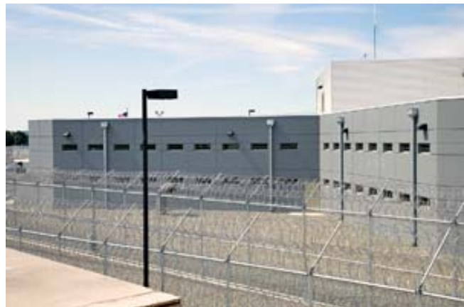
Monroe Correctional Complex's Intensive Management Unit received the first Silver rating for a prison facility housing unit in the country.
