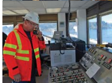
Tom Ford, bridge technician, operates the control panel to separate the bridge pontoons as a vessel transits the canal.
