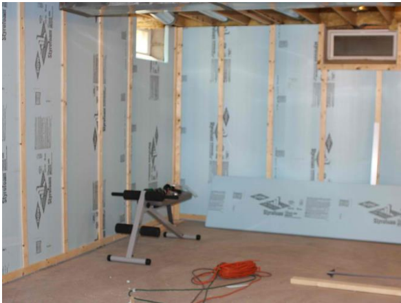
Interior insulation R-15 continuous
