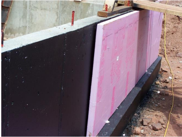
R402.2.8 Basement Walls Exterior insulation R-10 continuous
